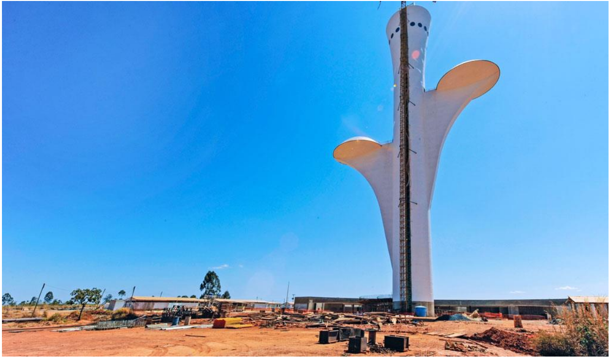
Digital TV tower construction in Brasilia, Brazil (photo: Wagner Santos/Avalon/Newscom)
