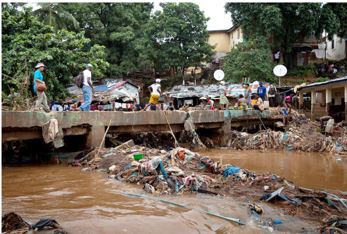
Indiscriminately dumped garbage and poor drainage systems.
