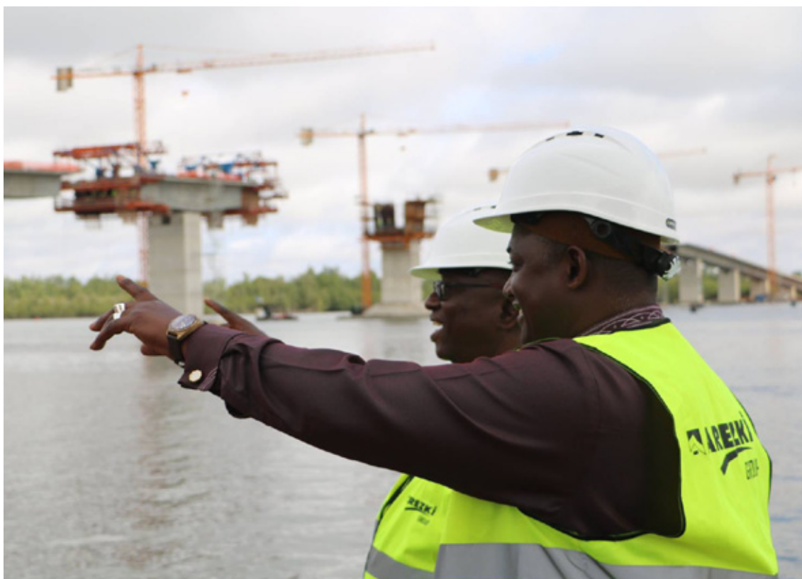
Large-scale infrastructure for sustainable development.
