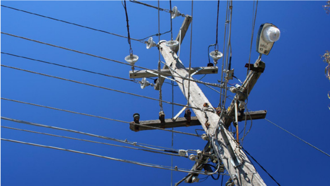
Existing infrastructure requires massive improvement.
