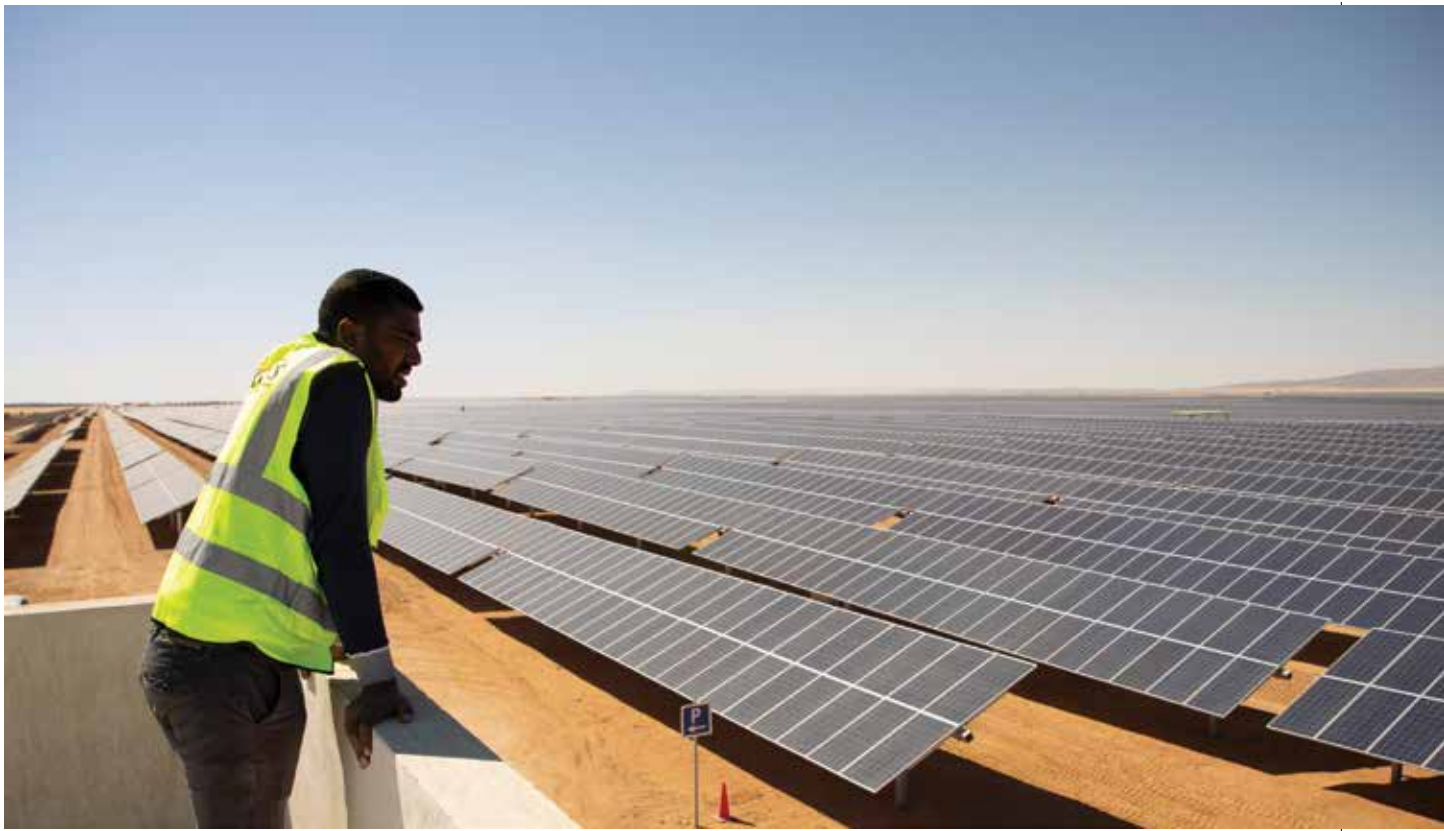
The Benban Solar Park in Benban, Egypt.
