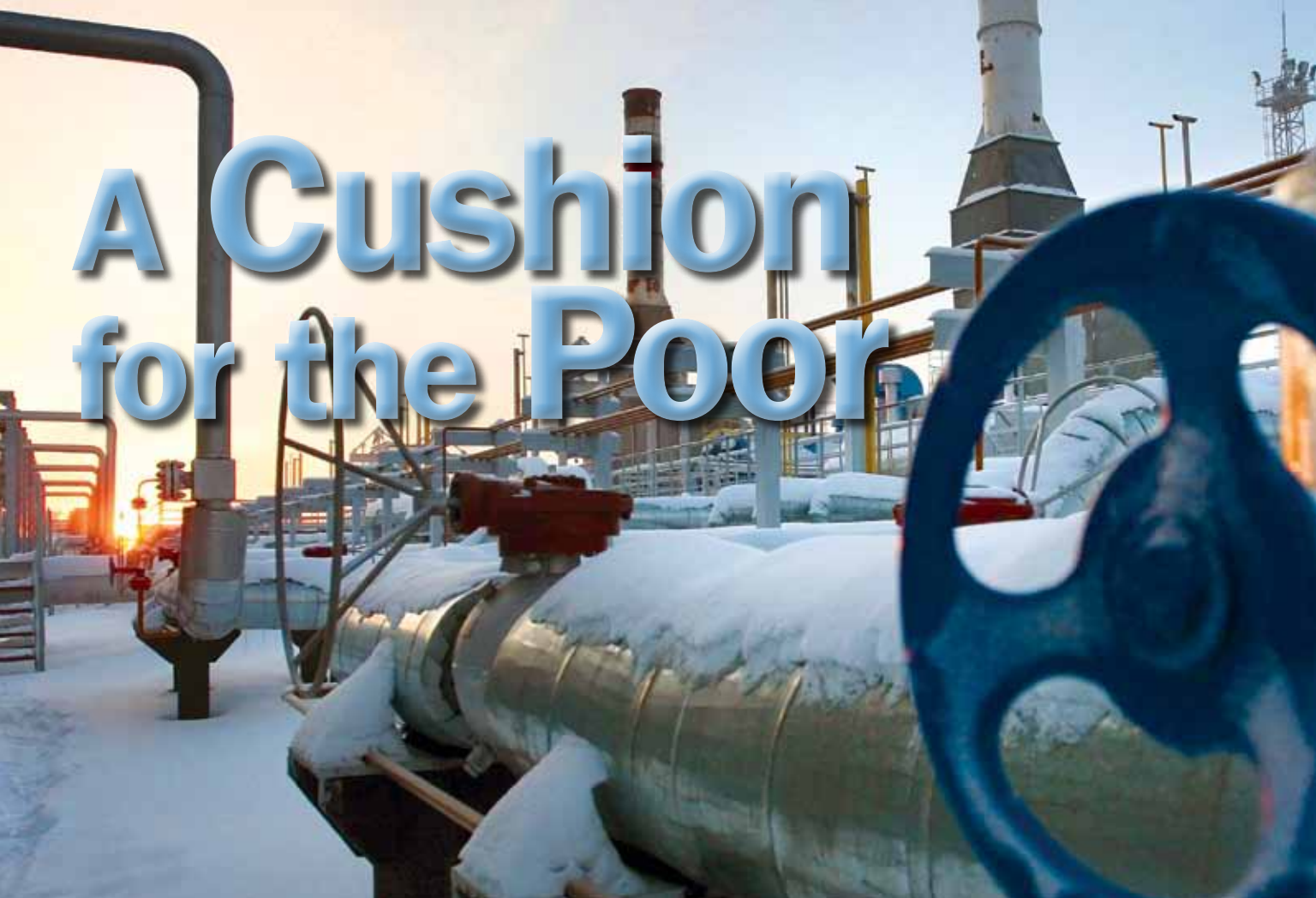
Oil and gas plant in Novy Urengoy, Russia.
