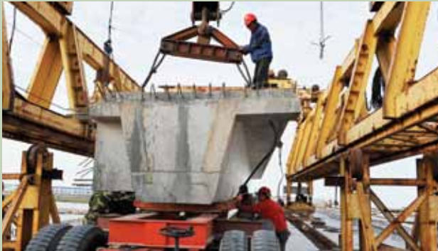
Construction project in Jiangsu, China.
